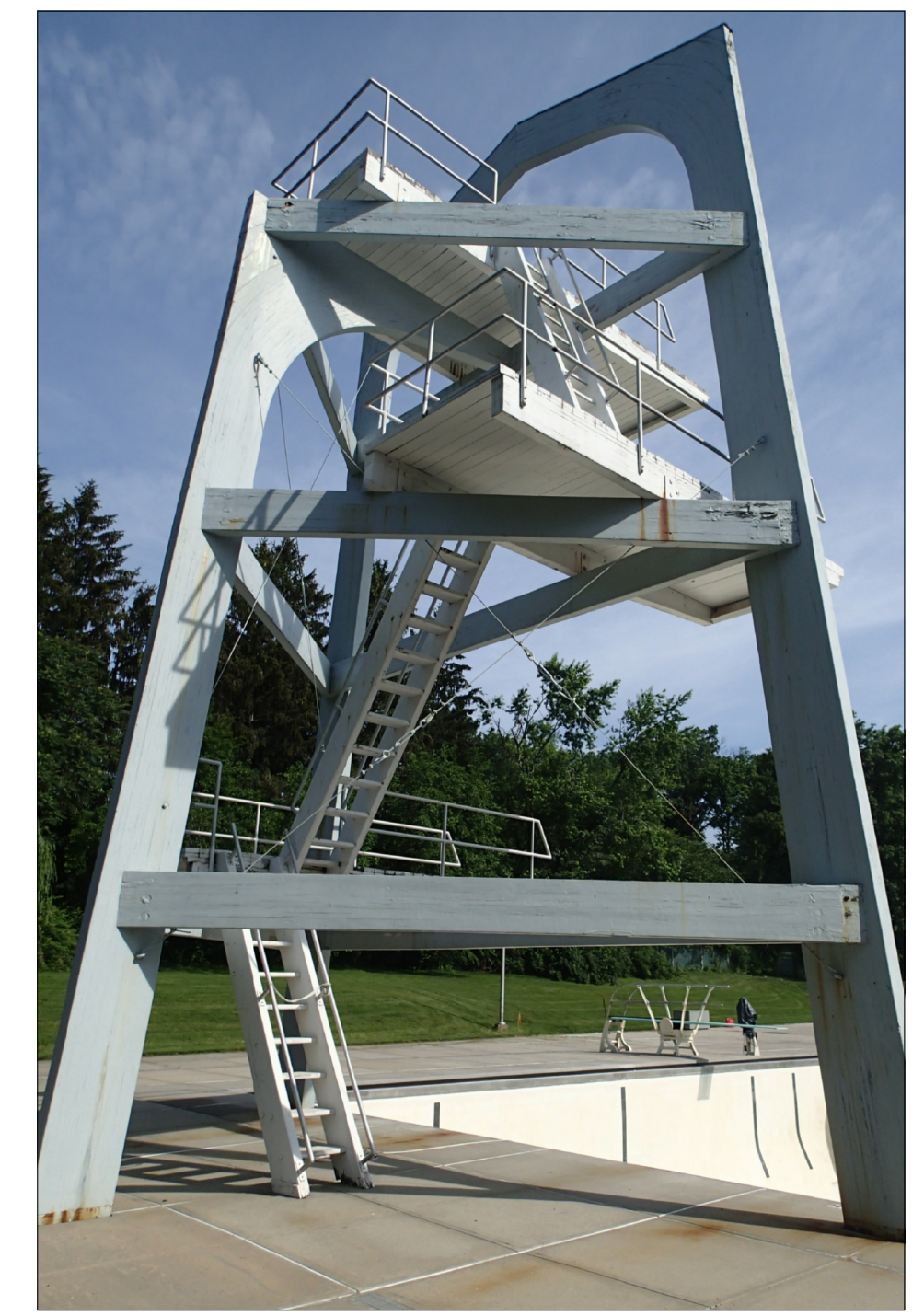
EXISTING DIVING PLATFORM STAND
